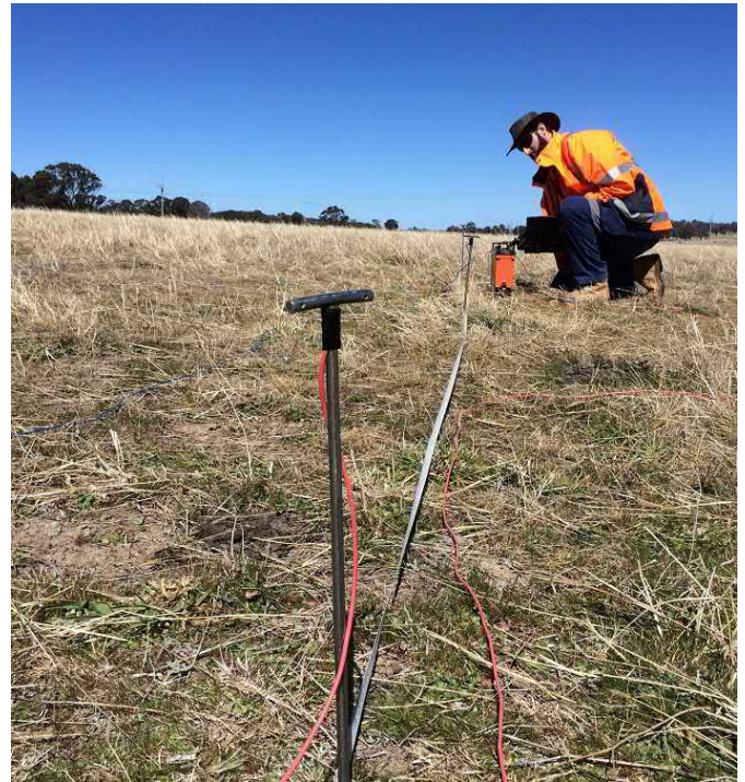
Fig 2: Typical setup for a geotechnical investigation
