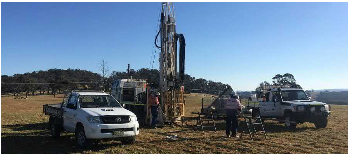
Fig 3: Typical setup for a geotechnical investigation
