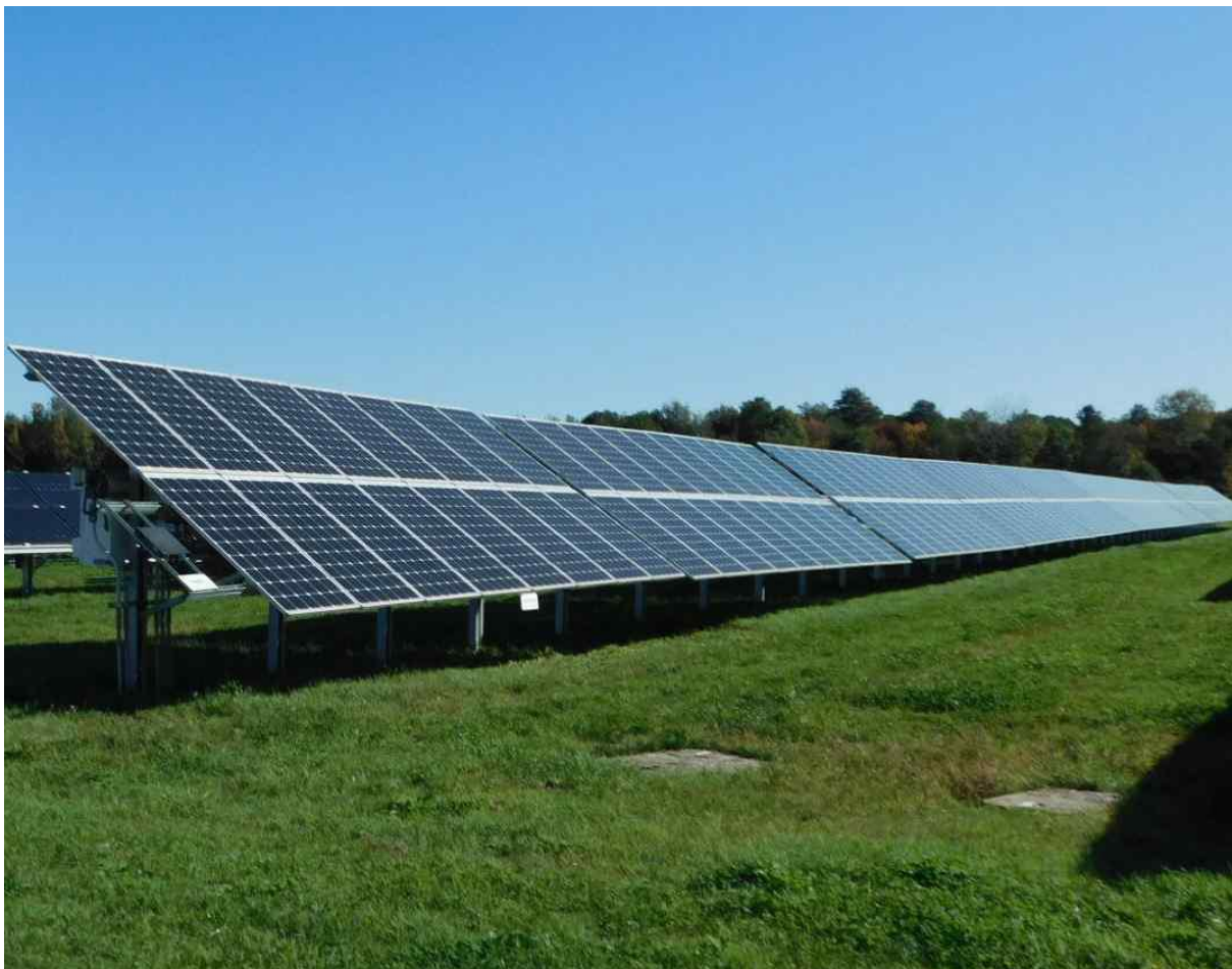
Figure 2.3: Typical single axis tracking system with two modules in portrait orientation (Supplied: South Energy)
